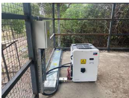
↑ 50 kWac SMA Inverter Installation
