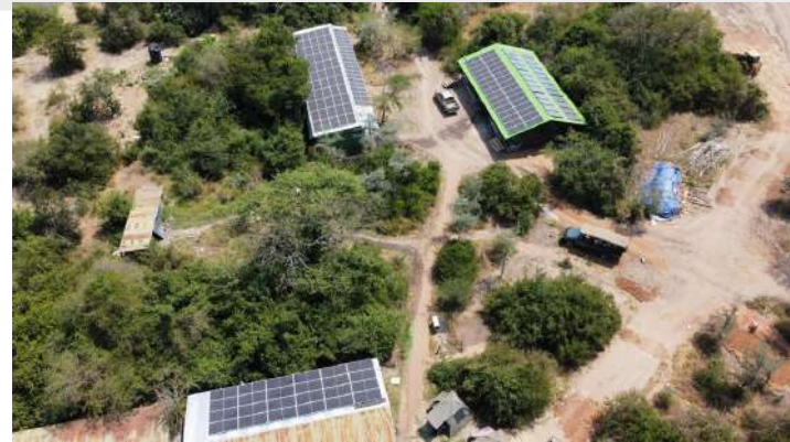
↑ 83.7 kWp Rooftop Solar Installation
