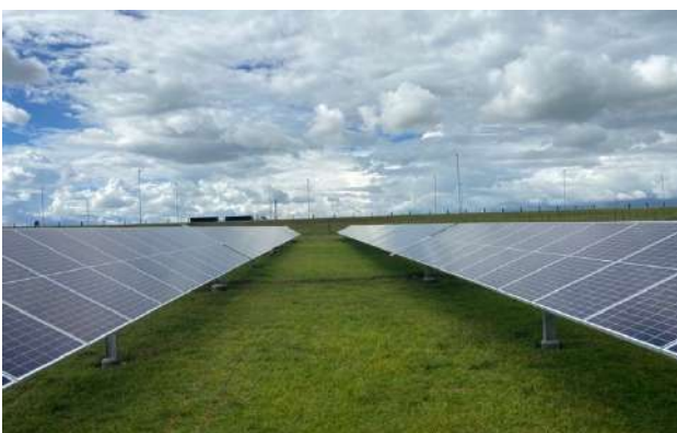
← Solar plant walkways for cleaners and technicians.
